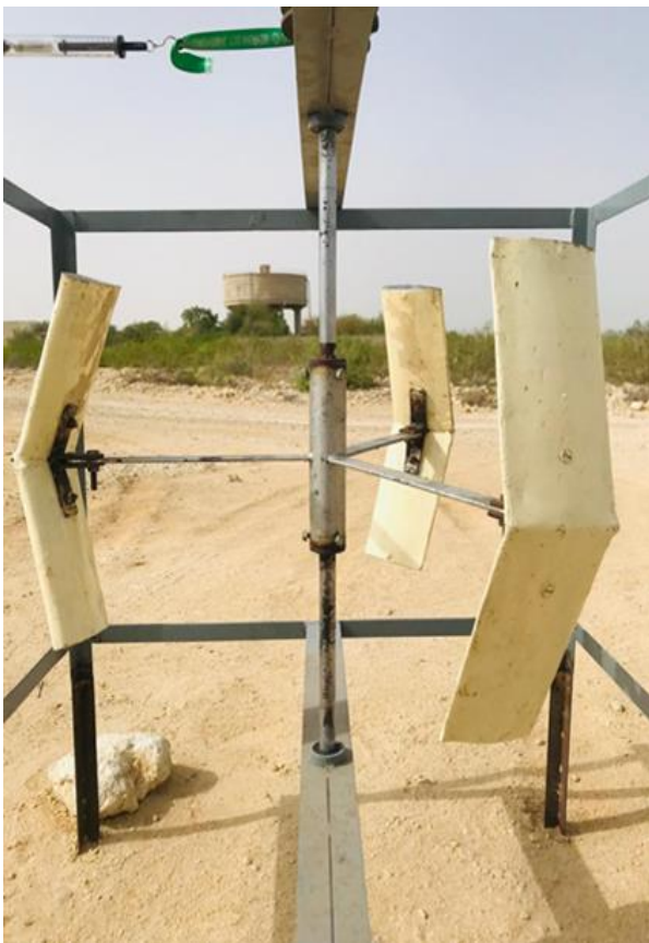
Figure.5. Assembly of the turbine
